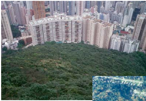
Rock fall hazards
