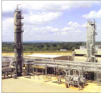
AES Shady Point Power Plant Captures 2-3% of CO 2 from a 320MWe CFB plant Panama, Oklahoma
