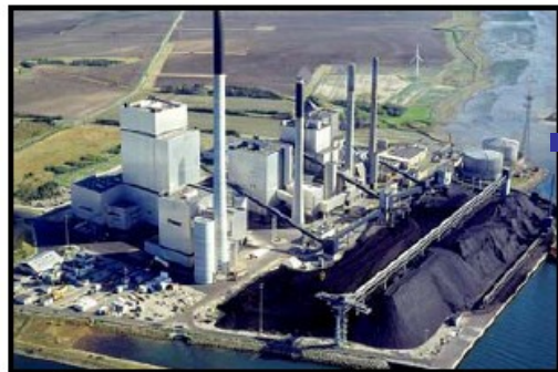
Capture compressed to 110 bar
