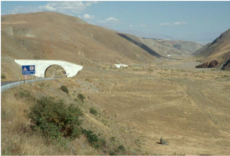
Three debris flow bridges in eastern Turkey, allowing debris flows from steep tributary valleys to cross a national road.
