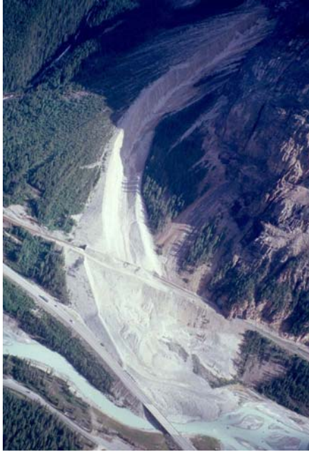
Mt. Stephen snow/debris shed, aerial view
