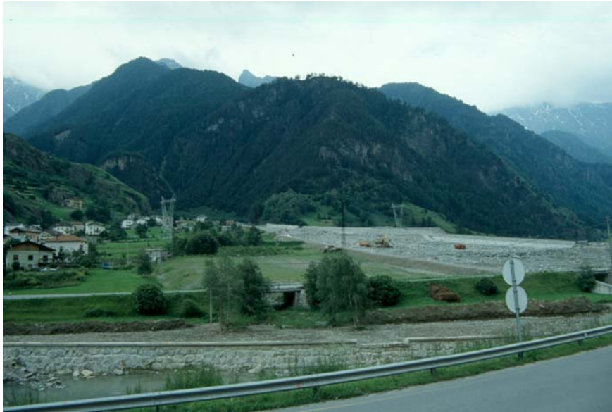
A segment of debris flow fan constrained by deflecting dykes, Arlberg, Austria.
