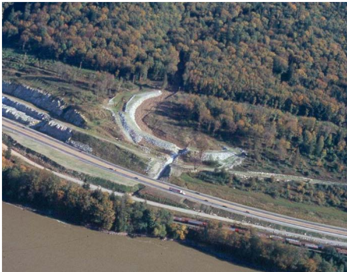
An open debris basin at Cheam View near Chilliwack, B.C. The brown material is the deposit of a debris flow retained by the basin. A low trash rack protects the outlet.
