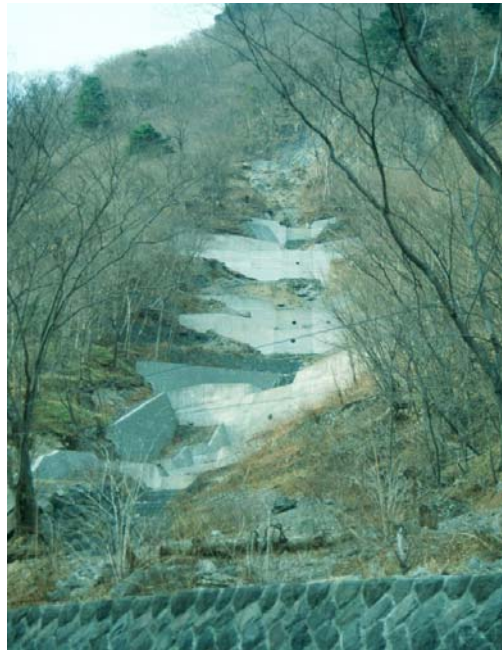
Check dams stabilizing a channel at Mt. Nantai-san, Honshu, Japan
