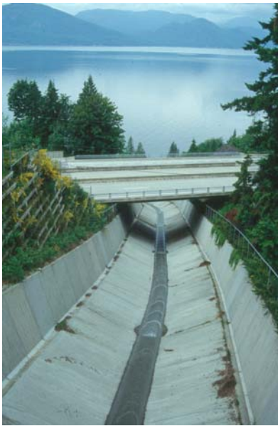
A lined channel designed for passage of debris flows on Alberta Creek, Lions' Bay, British Columbia
