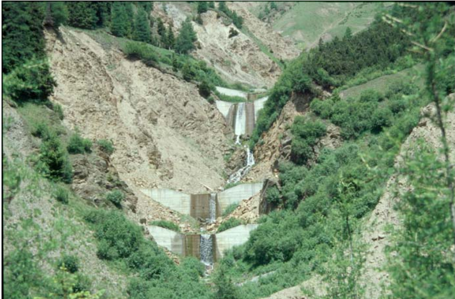
Check dams stabilizing a channel near Toblach, South Tirol, Italy.
