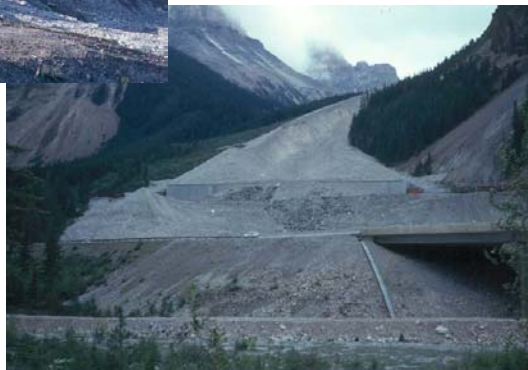
Mt. Stephen debris flow deposition area on the CP Rail main line, Kicking Horse Pass before and after the construction of a debris shed.
