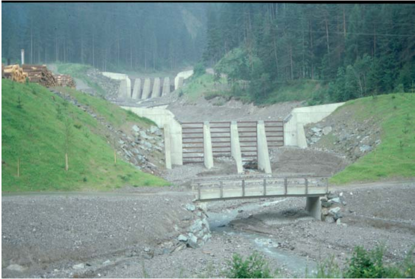
Two debris barriers near Lienz, Austria.
