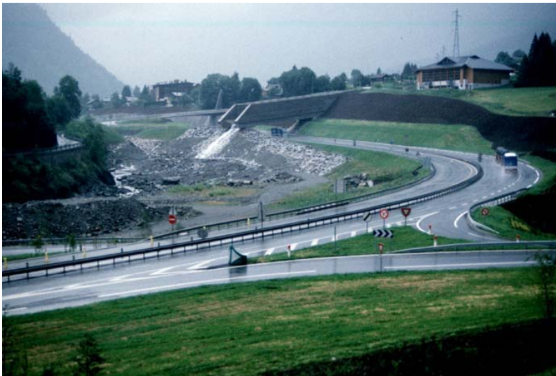
A debris flow bridge in the Savoy Alps, France
