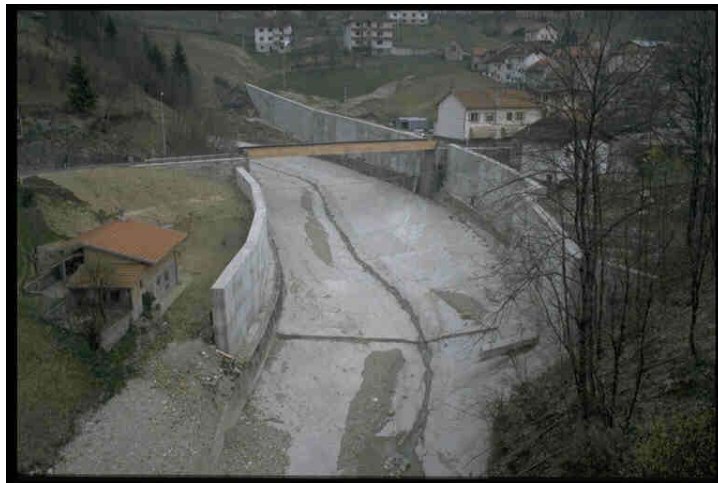
A channel conducting mud flows through the village of Lamosano, below the Tessina landslide, Northern Italy. The channel can be flushed by diverting water into it. (Photo by E. Bromhead, University of Kingston, UK.)
