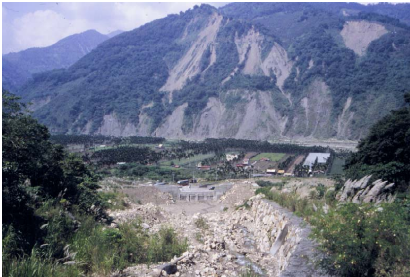
A debris flow barrier in Western Taiwan.
