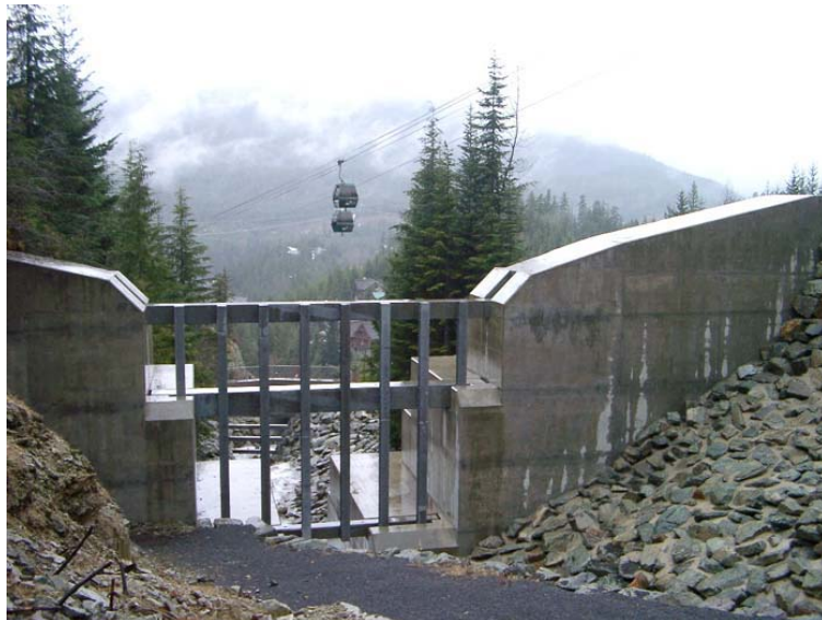
A debris barrier on Whistler Creek, Whistler, B.C., designed to retain 30000 m 3 of debris.
