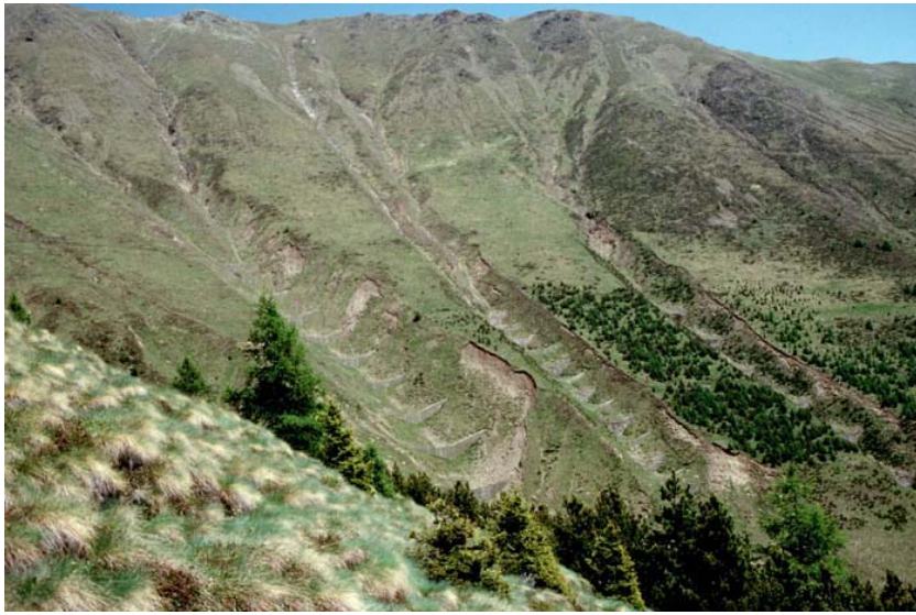
Check dams stabilizing the headwall of a watershed near Toblach, South Tirol, Italy.
