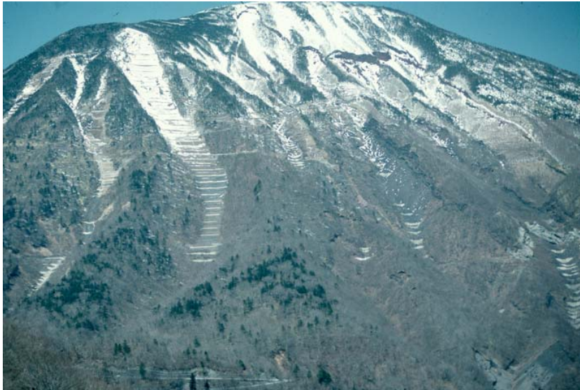
Check dams and erosion sills stabilizing a slope on Mt. Nantai-san, near Nikko, Japan.
