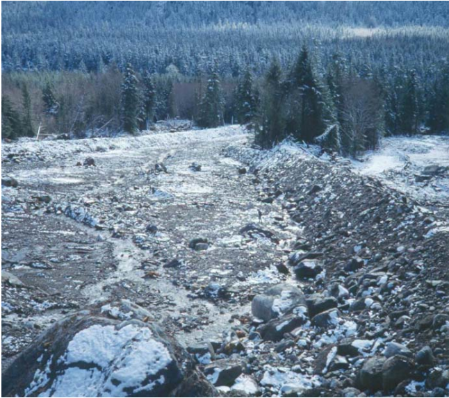
An open debris basin protecting the native village of Oweekeno, B.C. coast. Note figure near centre of photo for scale.
