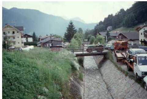
A "shooting channel" conducting a debris flow channel through the village of Matrei, Austria. The bridges can be lifted at the time of danger
