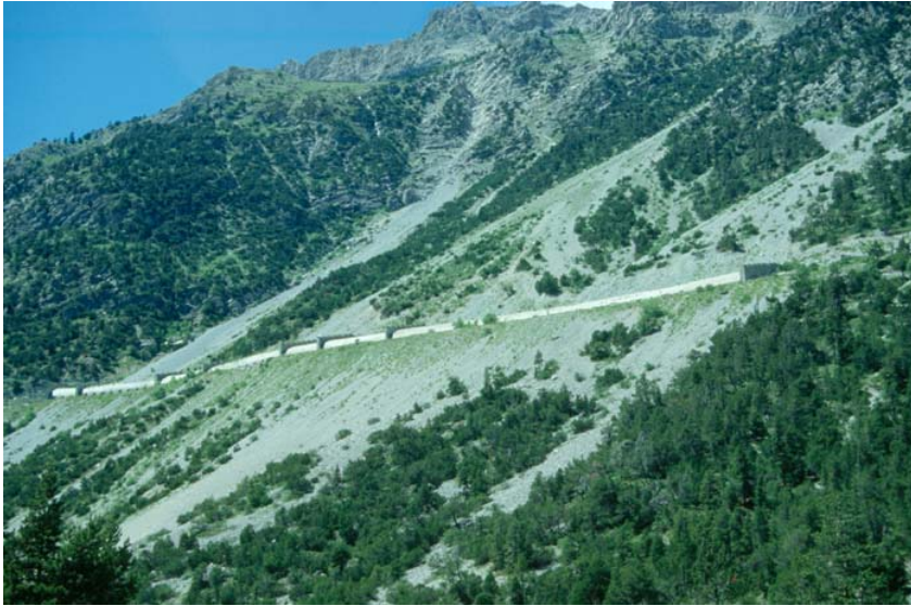
A long avalanche shed providing protection from rock fall and small debris flows on a talus slope, Switzerland.
